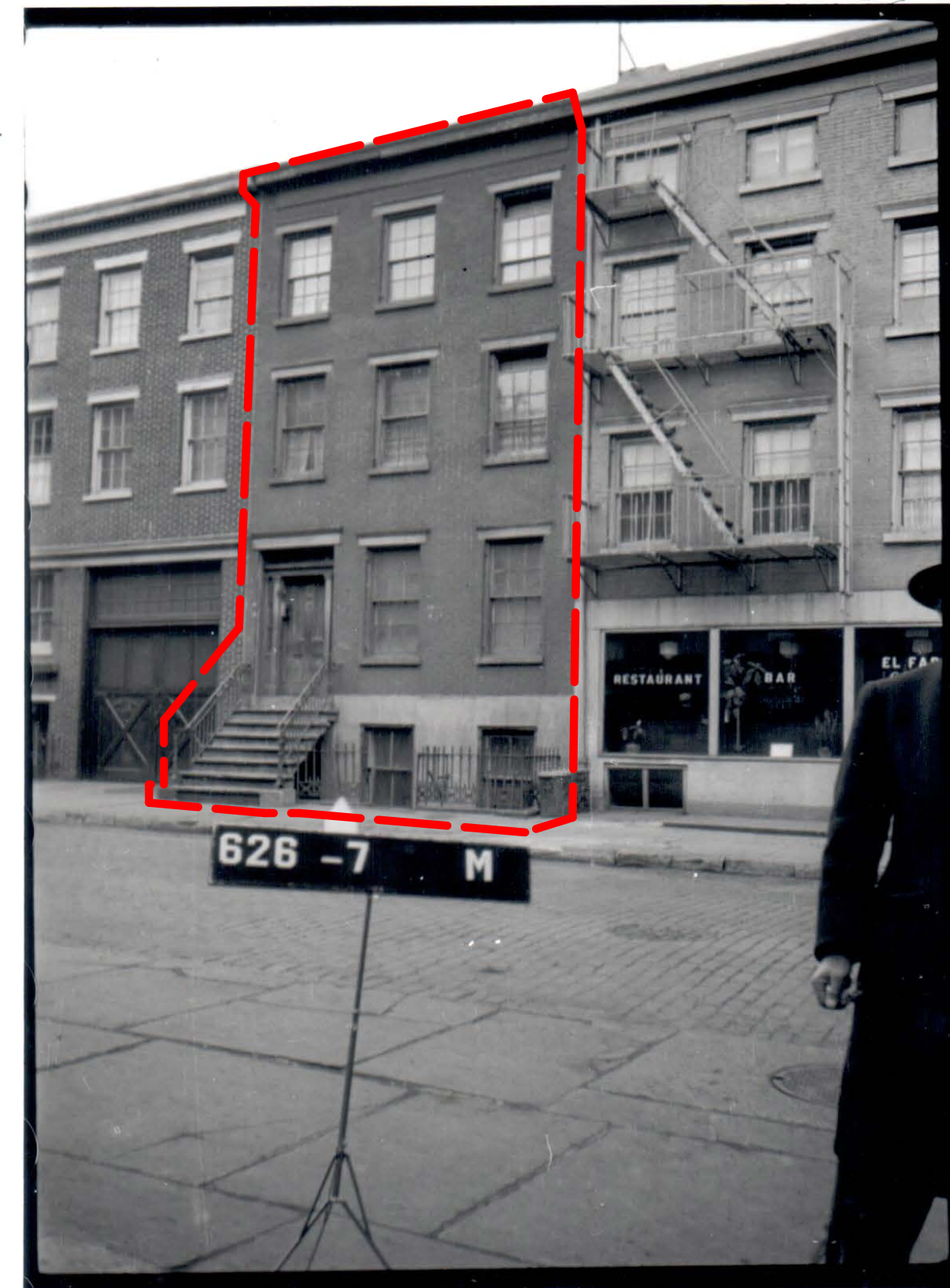
5 VIEW OF HORATIO STREET FAÇADE tax photo c.1940 NTS
